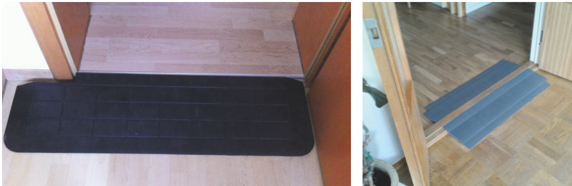
FIGURE 6: Examples of installed ramps to overcome door thresholds.
